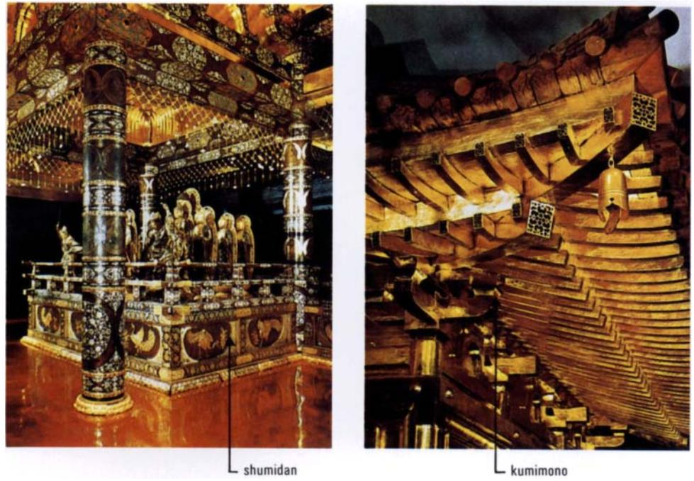
Figure 7. Chusonji Konjikido, showing typical architectural features.
